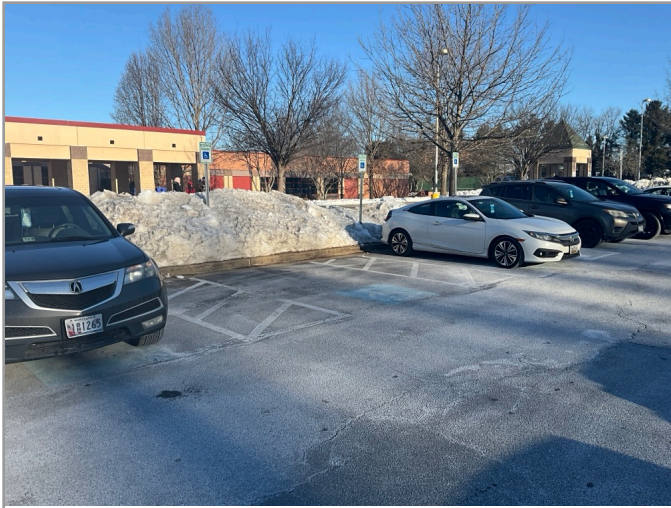
OVERVIEW OF ACCESSIBLE PARKING AREA
