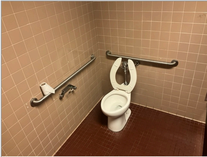
TOILET STALL OVERVIEW
