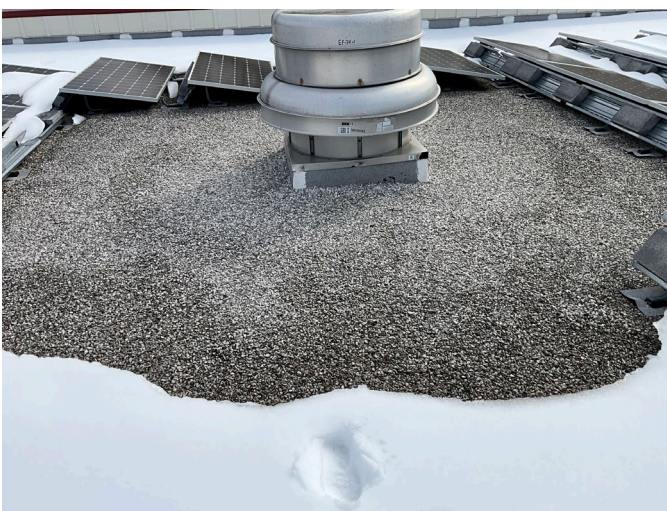
5 - PRIMARY ROOF OVERVIEW
